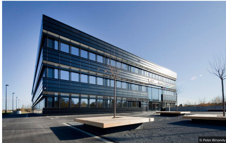
Figure 1.5: E.ON ERC Main Building
